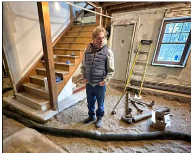
John Horchner surveys the basement flooring under construction. Photo by Nadine Horchner.
